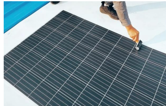
Install photovoltaic component
