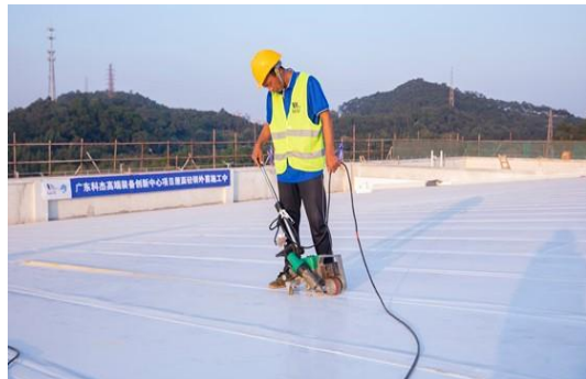
Weld the membrane
