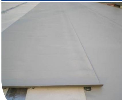
5、Install and weld waterproofing
