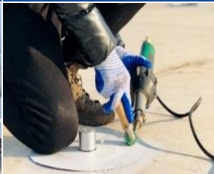
7、Install and weld base
