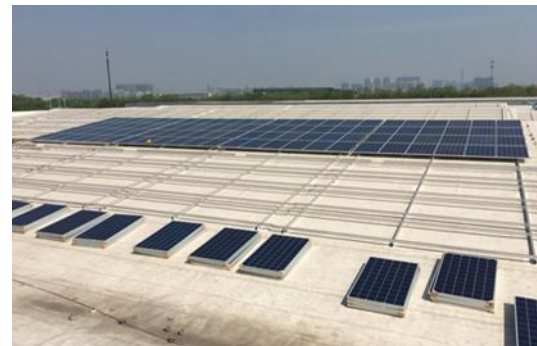
Install photovoltaic component
