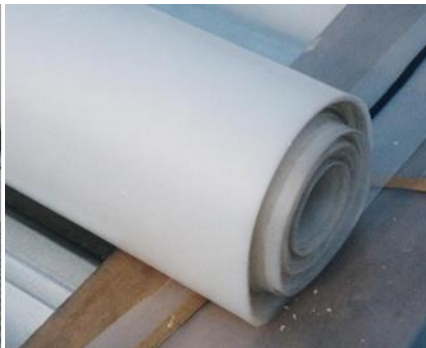
2、Install vapor barrier
