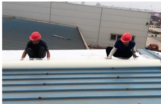
Install self adhesive TPO
