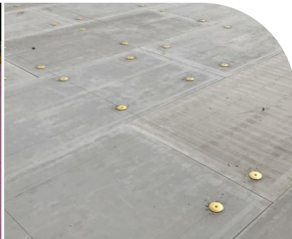
4、Install and fasten fireproof panel
