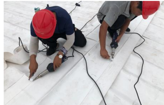
Weld the membrane
