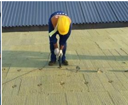
3、Install and fasten insulation
